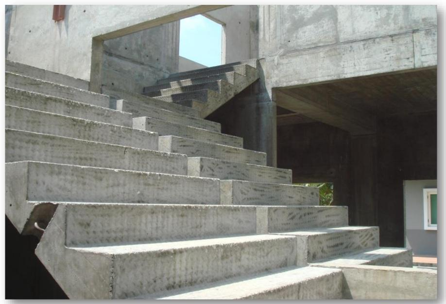
13.5a STAIRCASE 2 (in-situ landing slab support )
