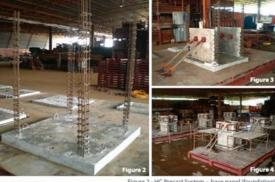
Figure 2 - HC Precast System – base panel (foundation) Figure 3 - HC Precast System - installation of ground floor wall panels Figure 4 - Completed 6 units of model for earthquake resistance test
