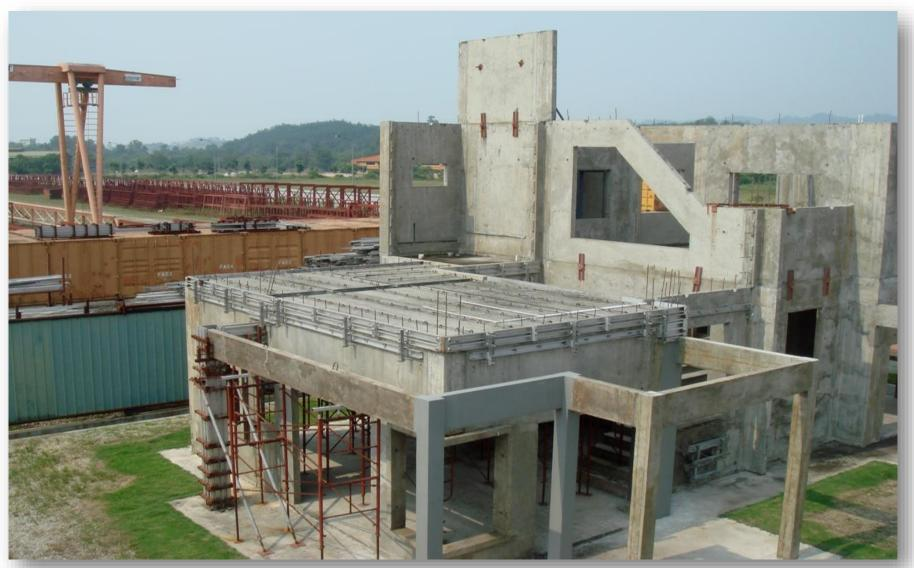
8 years exposed to weather, precast wall, staircase, half slab & beam with in-situ column.
